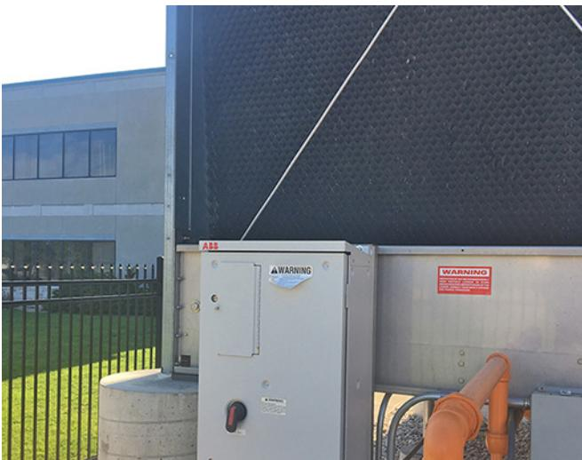
Using variable frequency drives (VFDs) with cooling tower fans can significantly reduce annual energy consumption in most climates, making them essential for projects focused on energy efficiency and LEED concepts.
