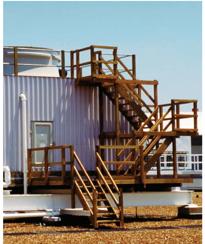
Wood Stairway with Access Platform
