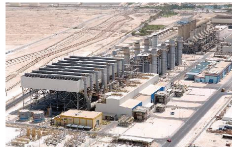
ALBA, Bahrain — ACC for 800 MW Combined Cycle Power Plant. A turnkey project.
