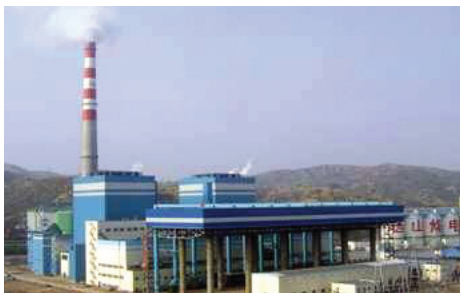
GUJIAO, China — ACC for 2x300 MW Coal Fired Power Plant.
