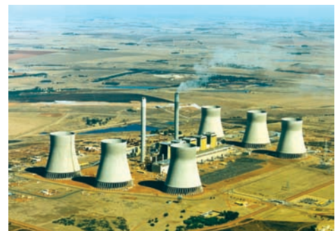
The world's largest Natural Draft Dry Cooling System - 6 x 690 MW Kendal Power Station, South Africa
