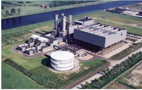
BRUGES, Belgium — ACC for 460 MW Combined Cycle Plant.
