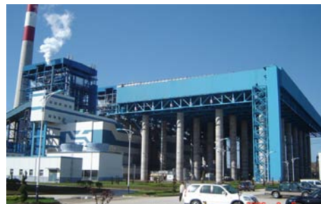
WUXIANG, China — ACC for 2x600 MW Coal Fired Power Plant.
