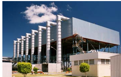
RIO BRAVO, Mexico — ACC for 3x515 MW Combined Cycle Power Plant.
