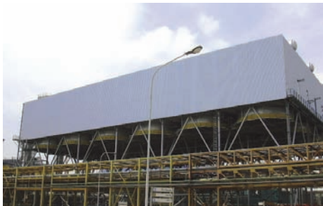
MANTOVA, Italy — 2x380 MW Combined Cycle Power Plant .
